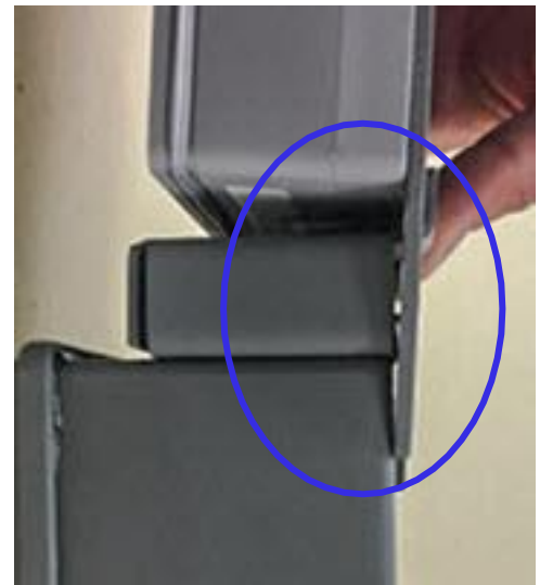
Figure 25: Check for gap between the top and base AMR mounting brackets
