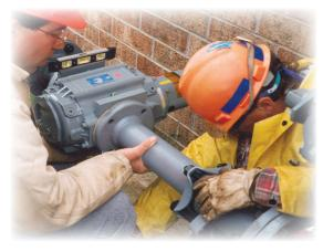
designed, manufactured and tested in accordance with API 1104 and DOT 192 to ensure system integrity with ROOTS precision engineered measurement products. This provides for fast, smooth, low-cost retrofit installation of high performance ROOTS rotary measurement products.
